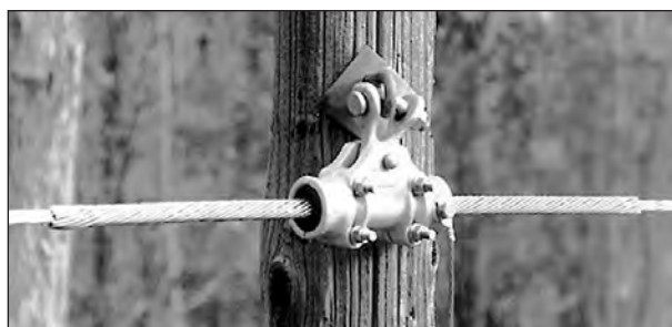
FIBERLIGN Cushion Clamp installed
